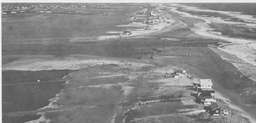
Westhampton Beach, N.Y. — View showing breakthrough barrier caused by 1962 storm.
