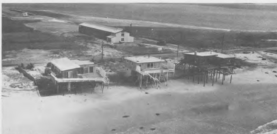
Westhampton Beach, N.Y. — View showing erosion around building foundations.
