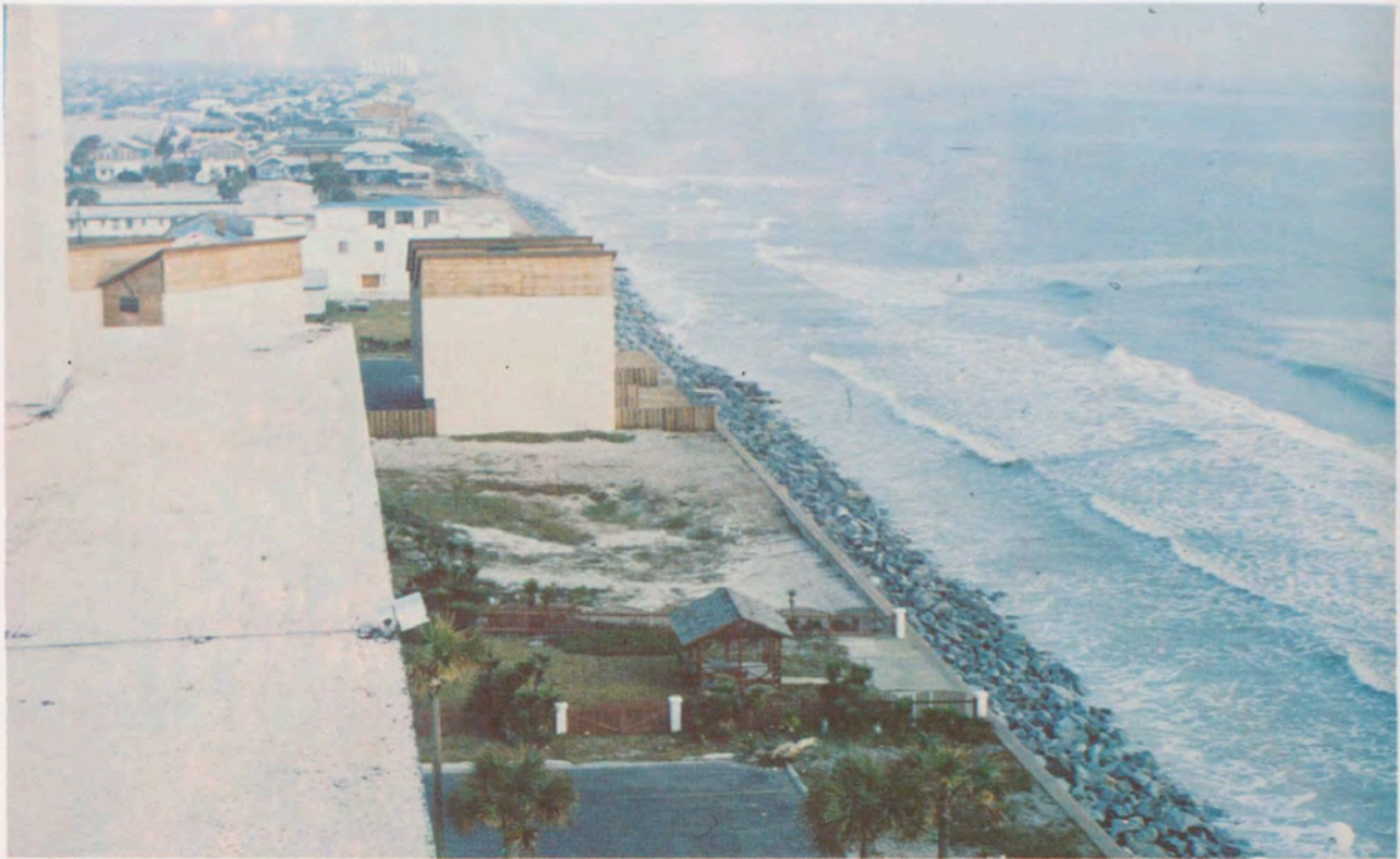
Eroded shoreline at Atlantic Beach (Duval County) before restoration.
