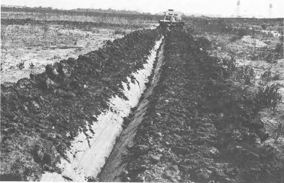
Figure 26. Trackmaster and drag plow trenching operation in progress
