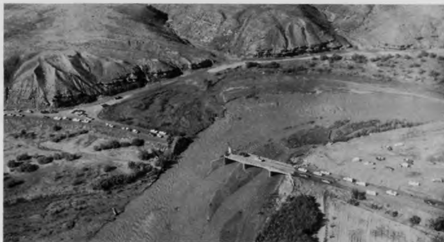
Right bank abutment of State Highway 262 Bridge over McElmo Creek at Aneth was washed away during flooding in September 1970. (Desert News photo—Reed Madsen)
