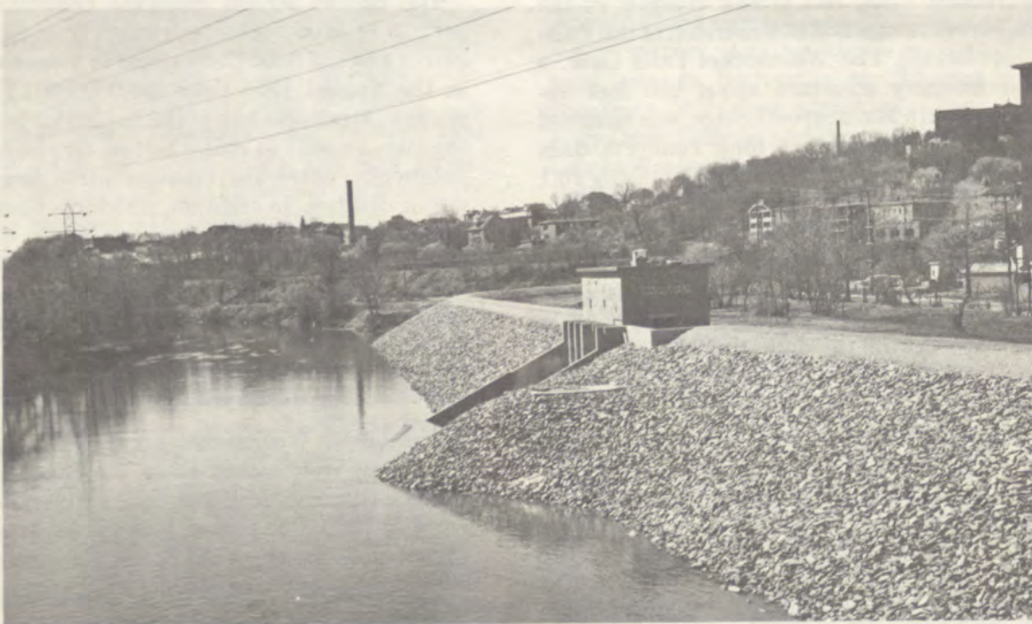
Lower Woonsocket Local Protection, looking downstream at Blackstone River dike and Hamlet pumping station
