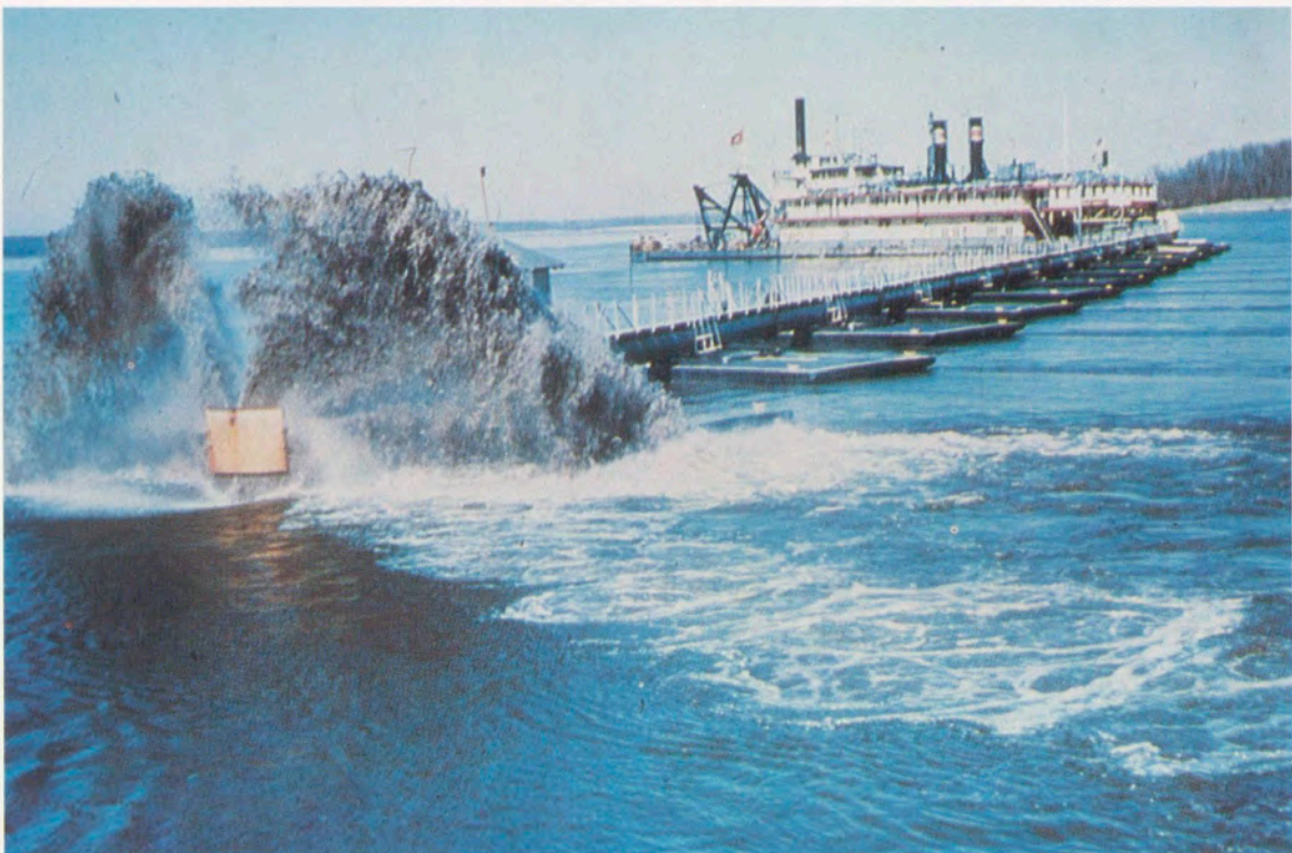
Dredging operations on the Mississippi River
