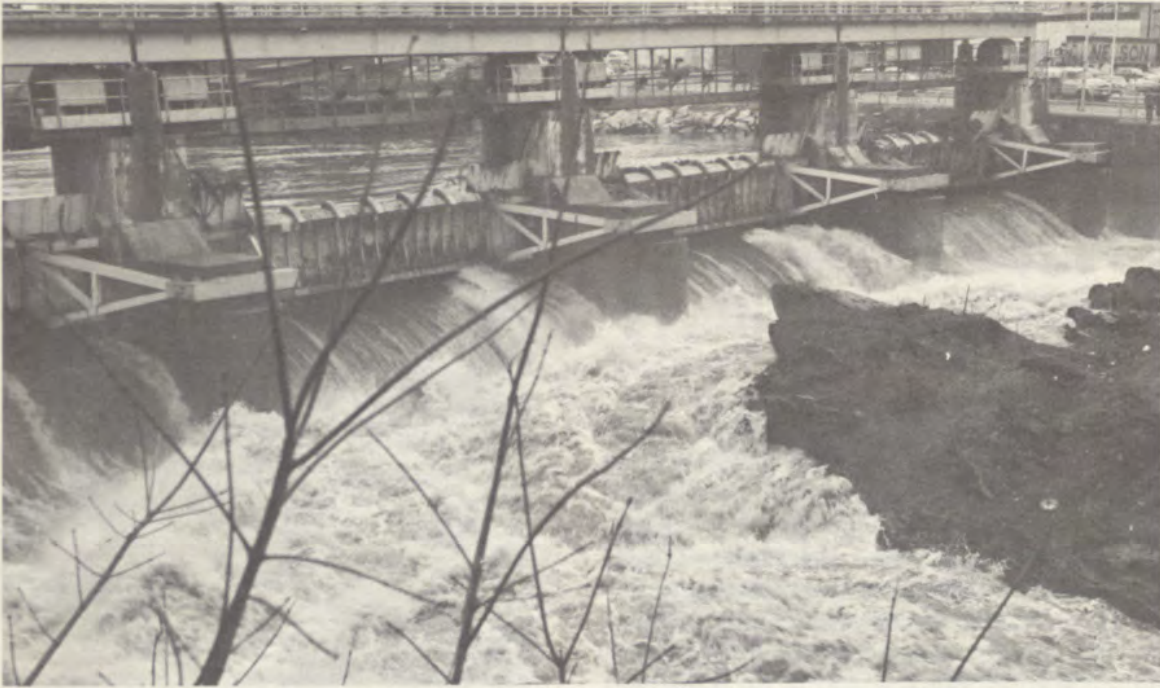
Woonsocket Local Protection, showing effectiveness of tainter gates to reconstructed Woonsocket Falls Dam in reducing river stages during March 1968 flood.
