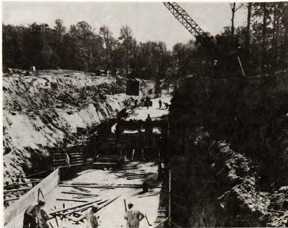
Figure 27. Pouring concrete for the bed of the 635-foot wave tank, 30 September 1949.
