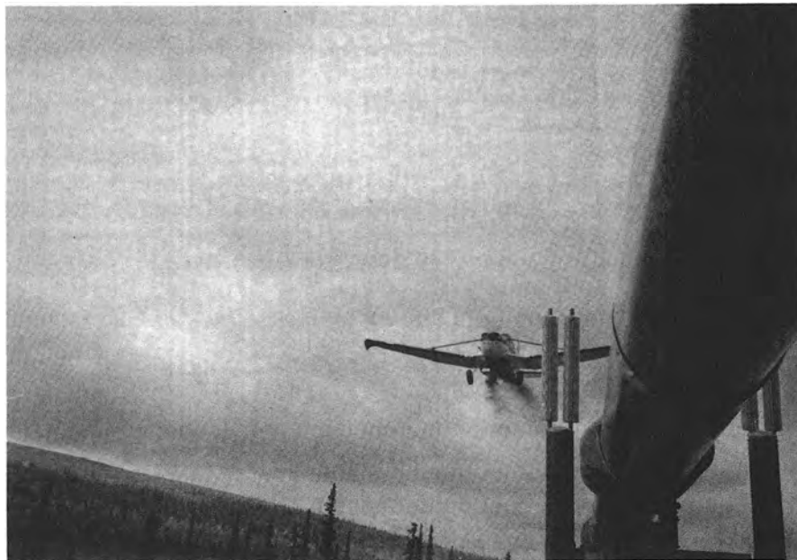
Figure 106. Aerial fertilizing of pipeline workpad in the vicinity of Old Man, September 1976.
