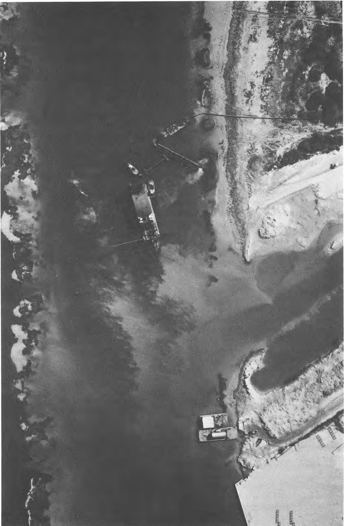
Figure 12. Turbidity creation by dredge plant equipment.
