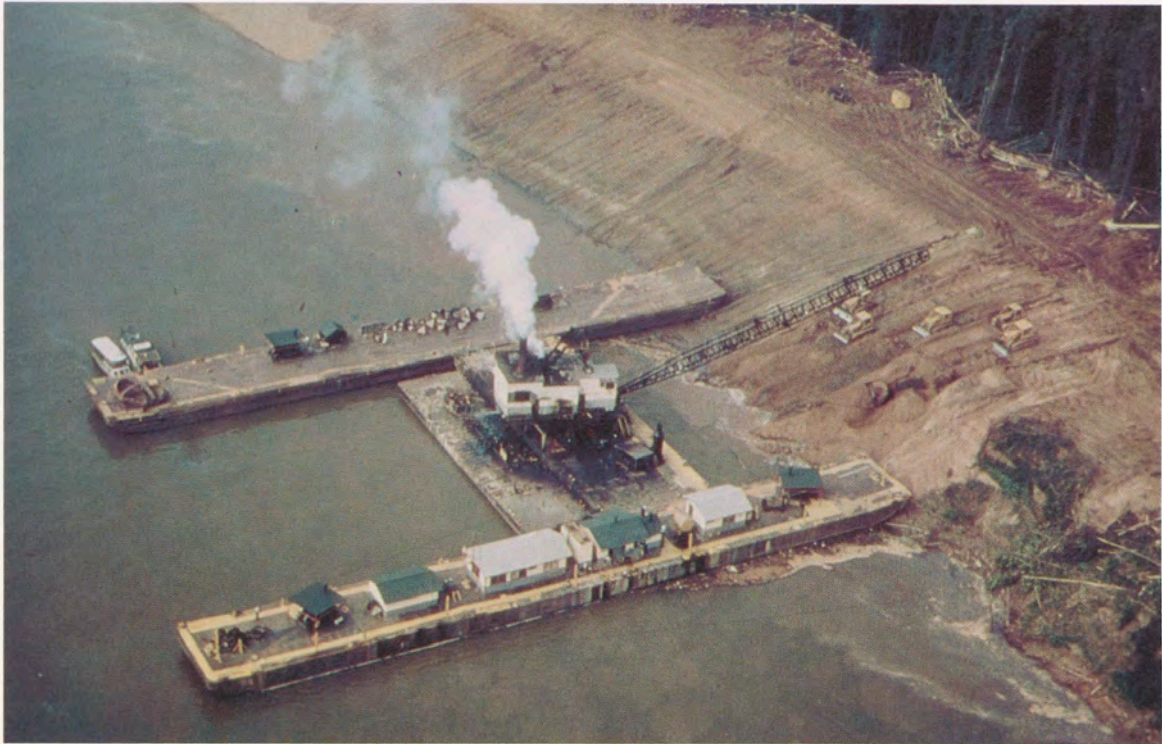
Bank grading for revetment work on the Mississippi River
